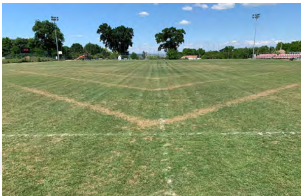
Poor drainage, leading to loss of grass cover
