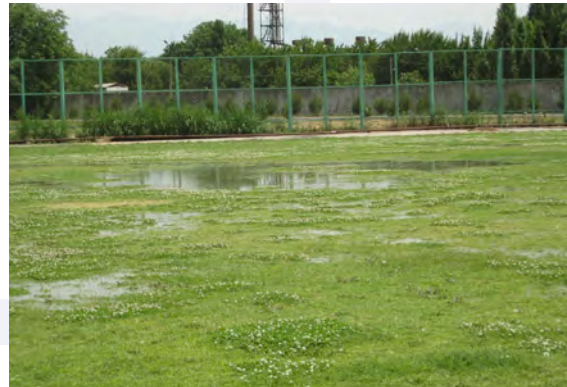
Poor surface levels, poor drainage and weed invasion
