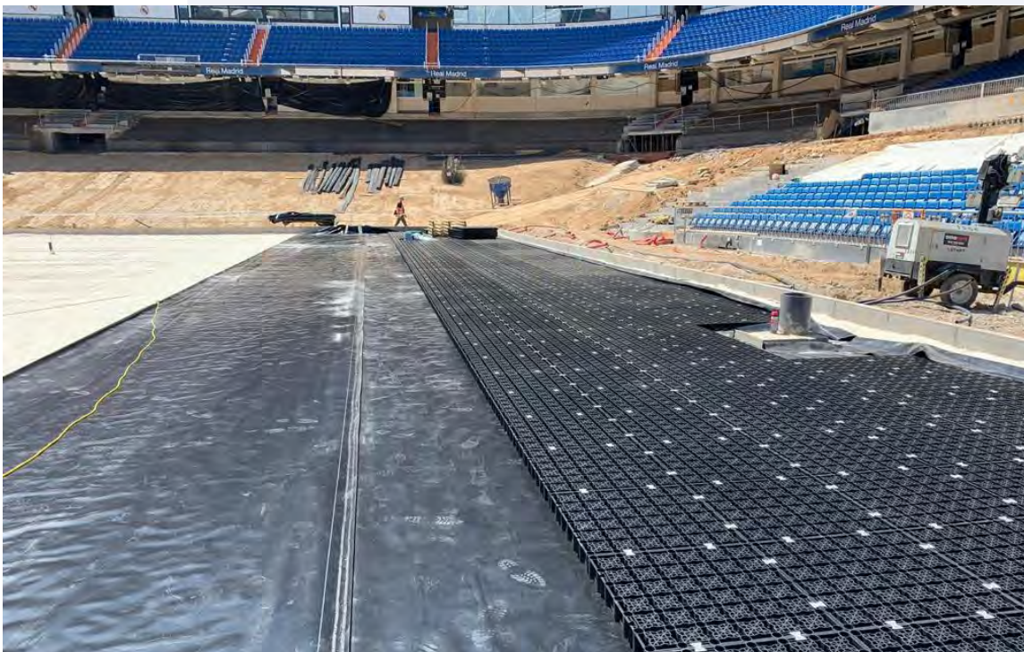
Figure 6: Plastic-reinforced egg-crate drainage system
