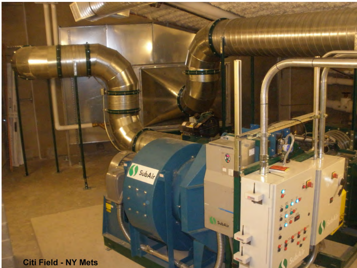
Figure 25: SubAir plant room installed within a stadium to operate the vacuum and ventilation system
