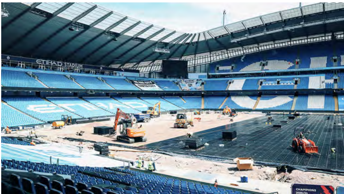
Figure 24: Vacuum and ventilation system with an egg-crate drainage base
