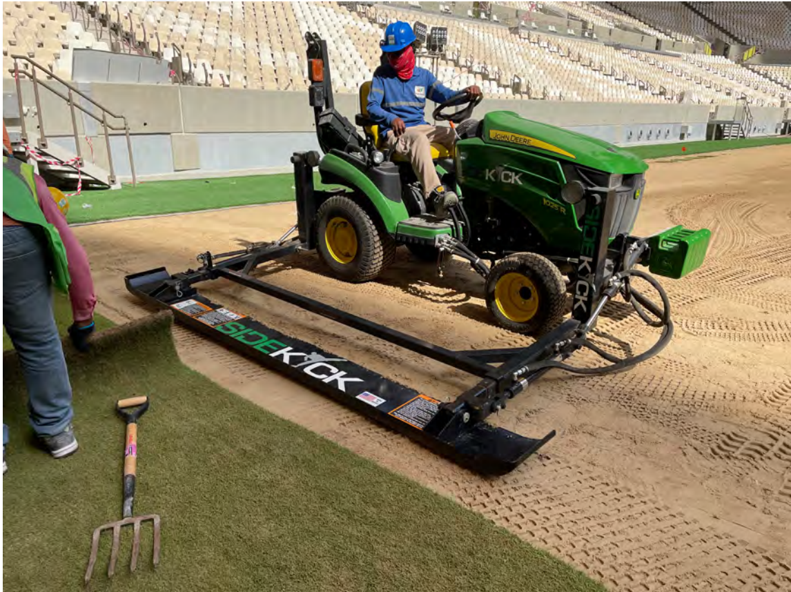
Figure 30: Push machine for turf lining
